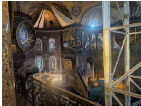
PLATE 74 Scaffolding under the dome.
